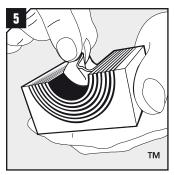
Adapt the module to the cable size. Peel off layers until you achieve the gap seen in picture 6. The halves may not differ by more than one layer.
